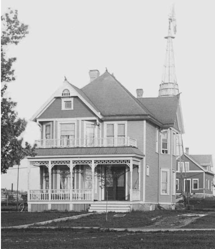
This shows the Larson House in its early days - notice the windmill for bringing up water from the backyard well and the railroad materials along the tracks.
