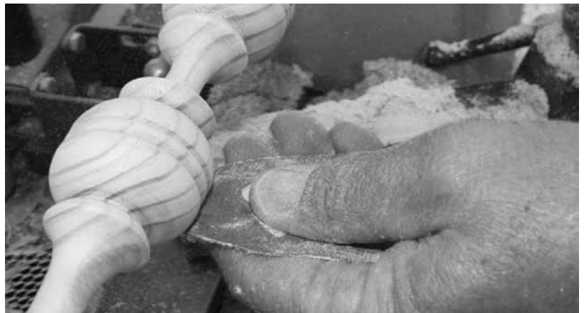
Sanding a new spindle to replace a rotted one for the front porch. Below: A Christmas party at the Larson House.
