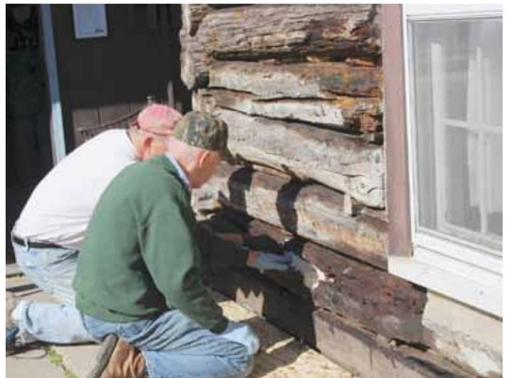
*Rod Clark and Dale Marsden apply epoxy wood filler to gaps in the logs.*
