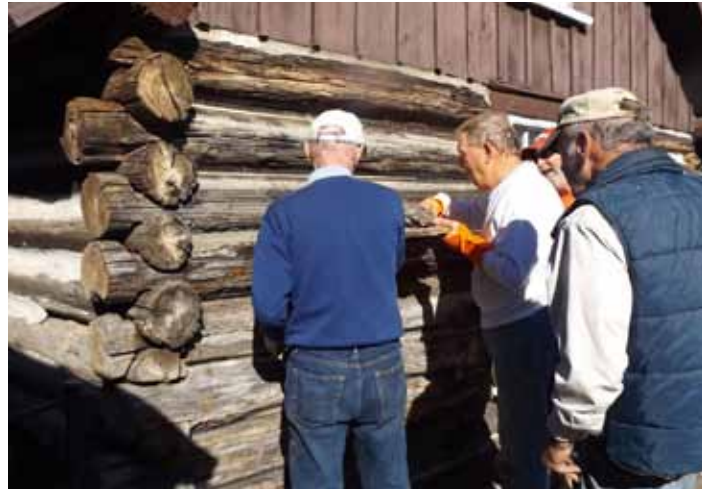
Dale Marsden and Rod Clark fill cracks as Joe Larson and Bob-Kolek look on. Joe and Bob prepared the wire and mortar.
